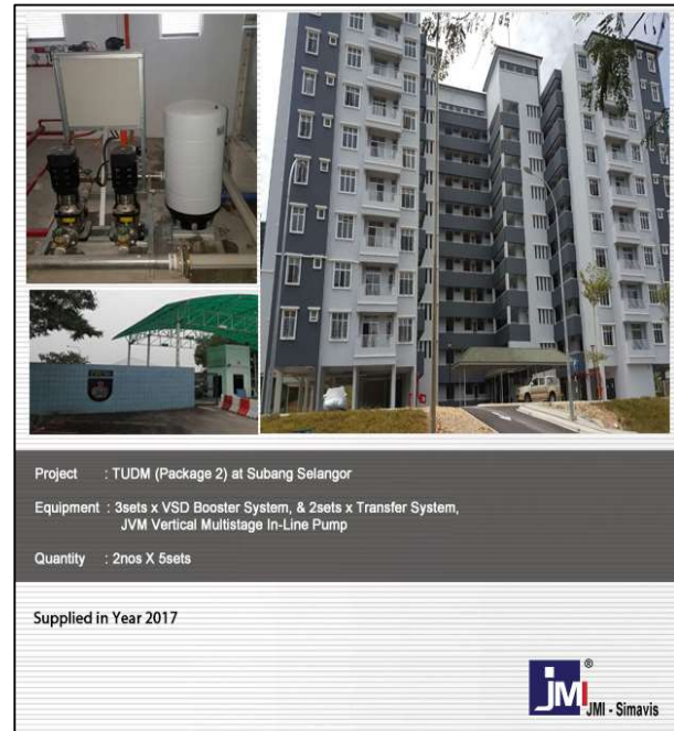
Year 2017 – VSD Booster & Transfer (6 sets) At TUDM (Pckg 2) Subang Selangor
