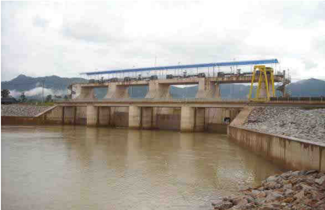
Besut Barrage (12m x 5.7m)
