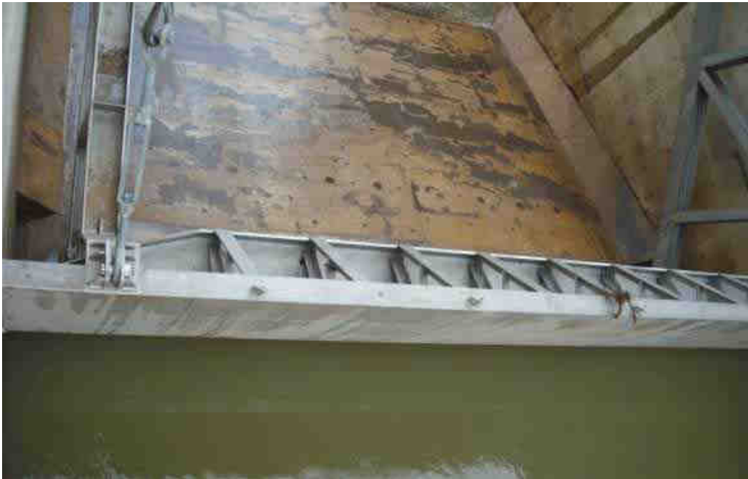
Testing Radial Gate for leakages
