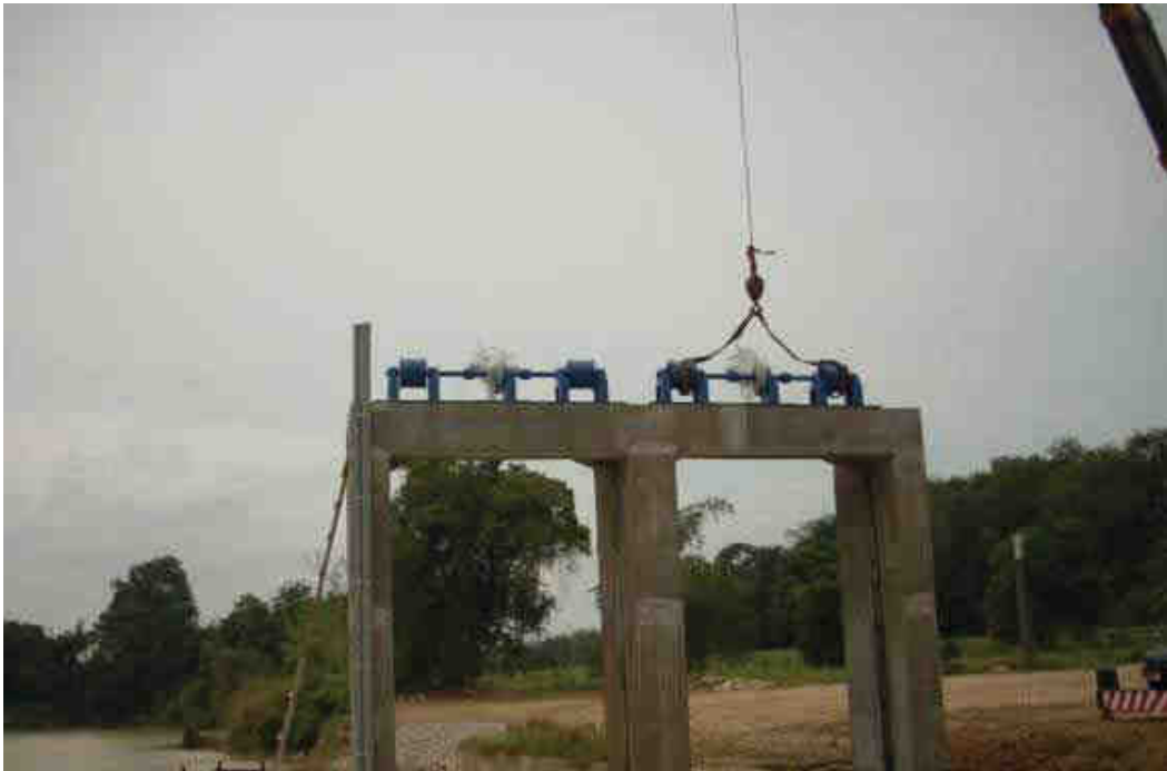
Hoist system for Roller Gates
