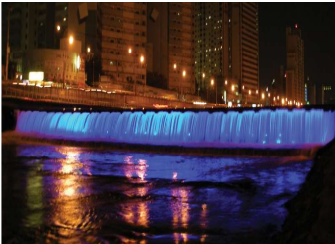
Night View of Crest Gate with Rubber Dam
