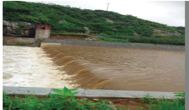
Inflation of Crest Gate with Rubber Dam
