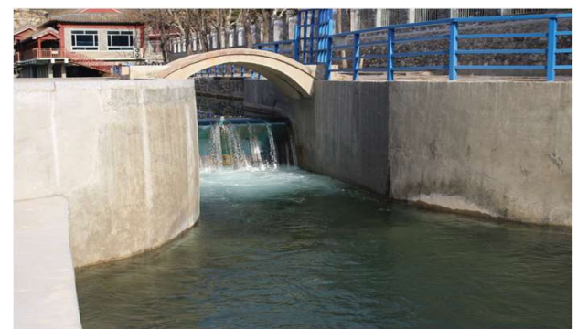
Beijing Fangshan Juma River Spillway Gate (2) 3.0m(H) x 2.3m(L)
