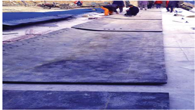
Installation of Inflatable Rubber Dam
