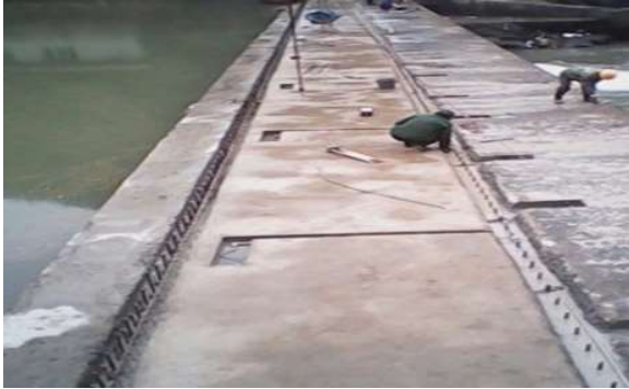
Installation of Anchor Bolt & Clamping Plate
