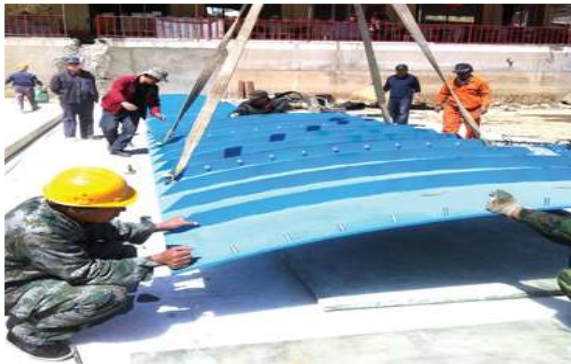
Installation of Crest Gate Panels
