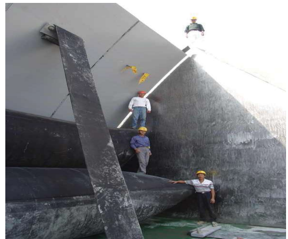
Crest Gate with Double Rubber Dam
